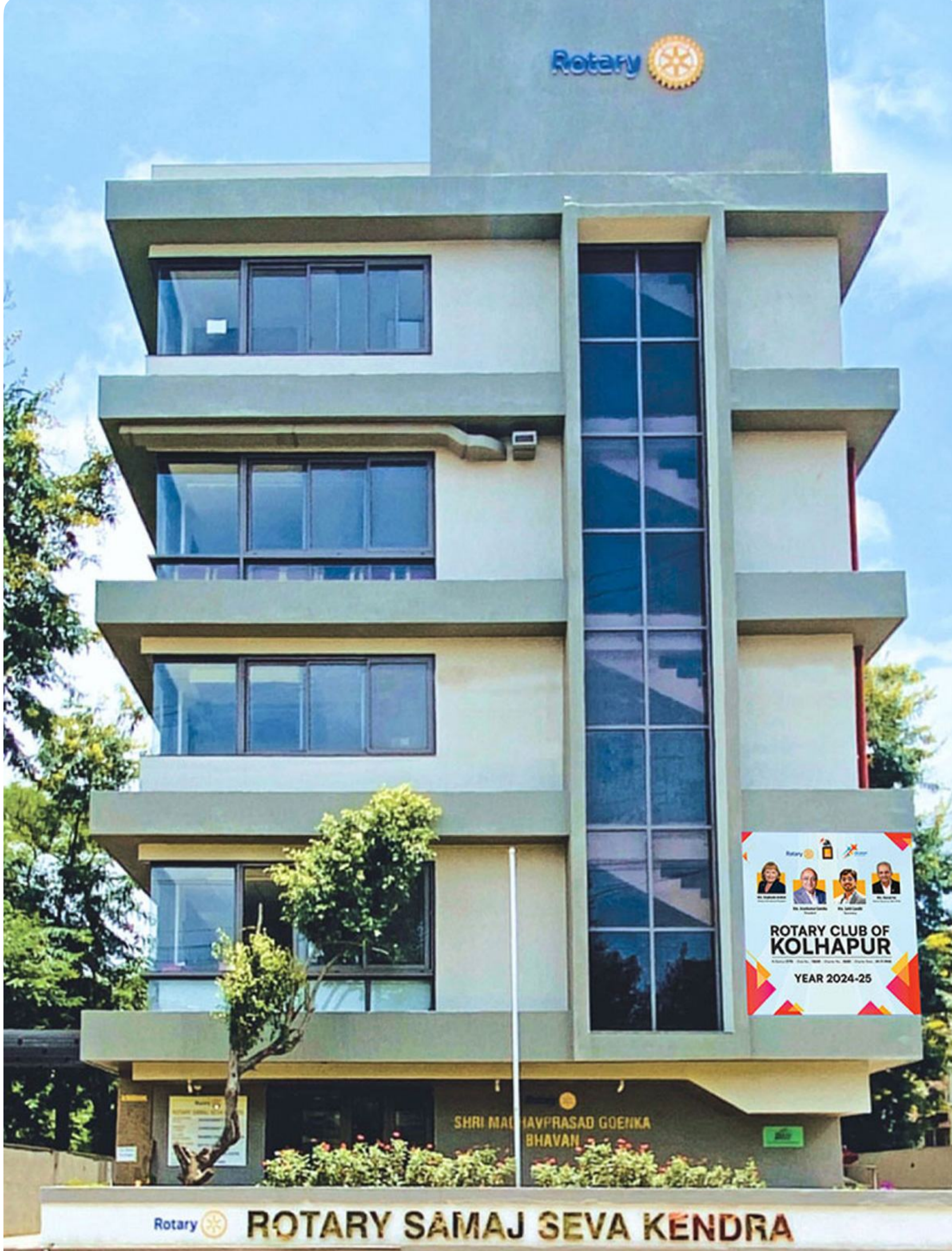
ROTARY CLUB OF KOLHAPUR'S ROTARY SAMAJ SEVA KENDRA BUILDING
